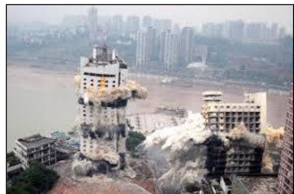
Fig. 13: Controlled Demolition of structures
