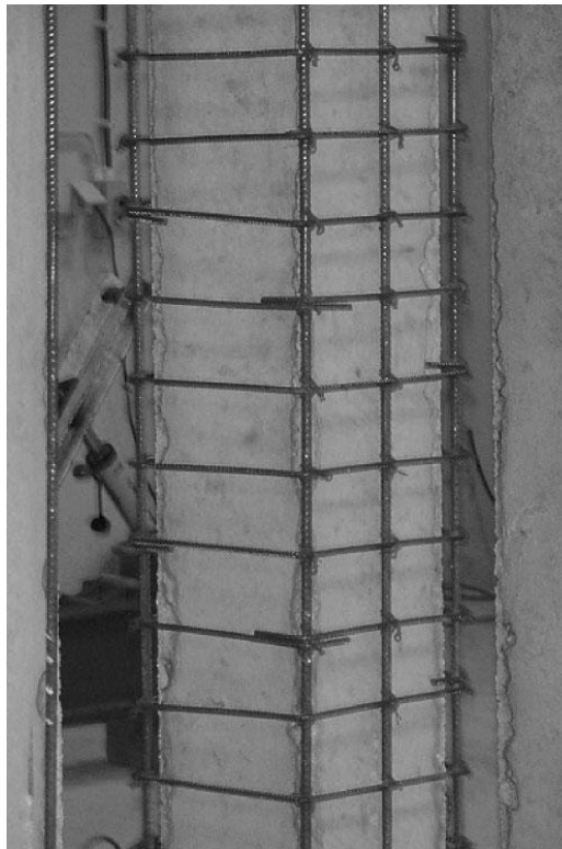
Fig. 27: Concrete Jacketing of RC columns
