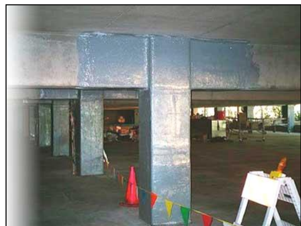
Fig. 26: CFRP wrapped column
