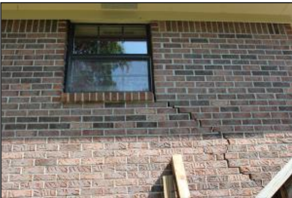
Fig. 5: (a) Sinking or Sloping floors, (b) Cracks in brick and block, (c) Foundation wall cracks, (d) Wall rotation, (e) Cracked or Bowing Walls, (f) Cracked floors, (g) Separation of windows from house, (h) Walls separating from house
