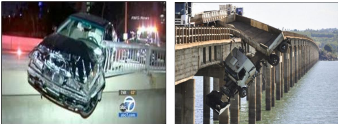
Fig. 9: Railing crash involving (a) smaller vehicle, (b) larger vehicle
