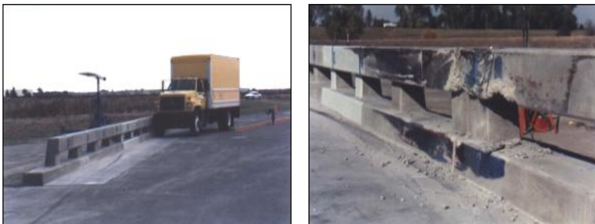
Fig. 10: Arrangements for vehicular-impact test of RC railings
