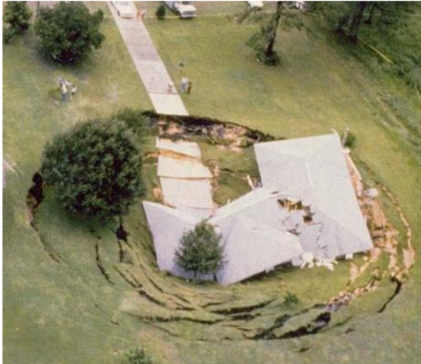
Fig. 4: (a) Sinking of entire structure due to support settlement
