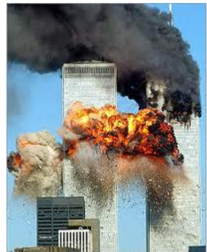
Fig. 12: Blast load on World Trade Center (September 11, 2001)
