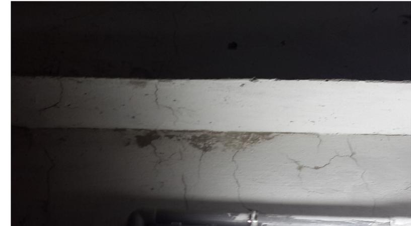
Fig. 6. Cracks in a beam in an AC plant of a spinning mill
