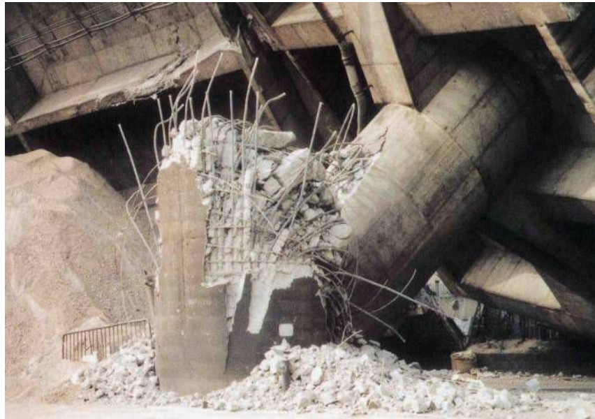
Collapse of the Hanshin expressway in the 1995 Kobe earthquake
