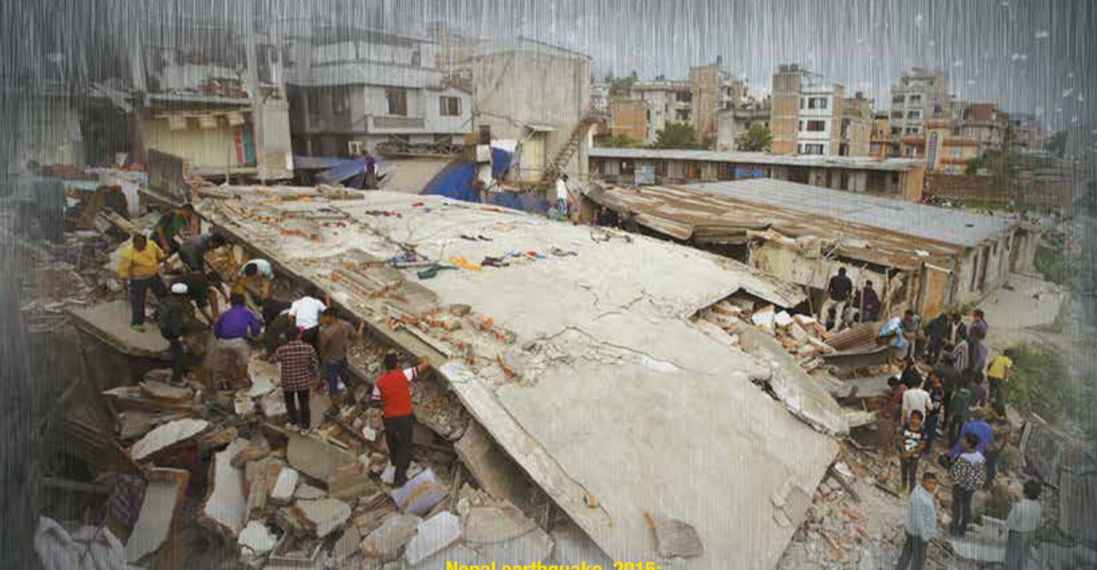
Nepal earthquake, 2015: Even single-story structures collapsed, killing all the occupants, as the structures were not built to resist earthquakes.
